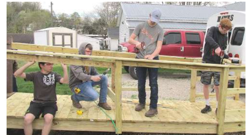
Trade students constructing an access ramp
