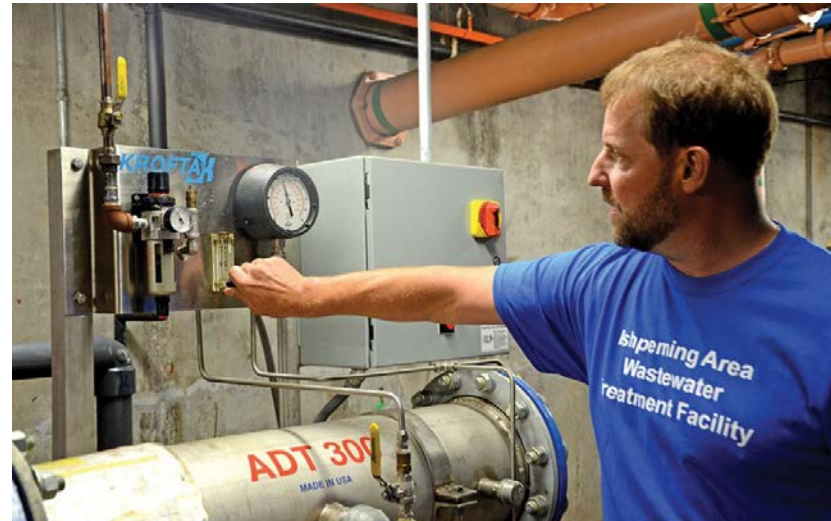
The Ishpeming Area Wastewater Treatment Facility
