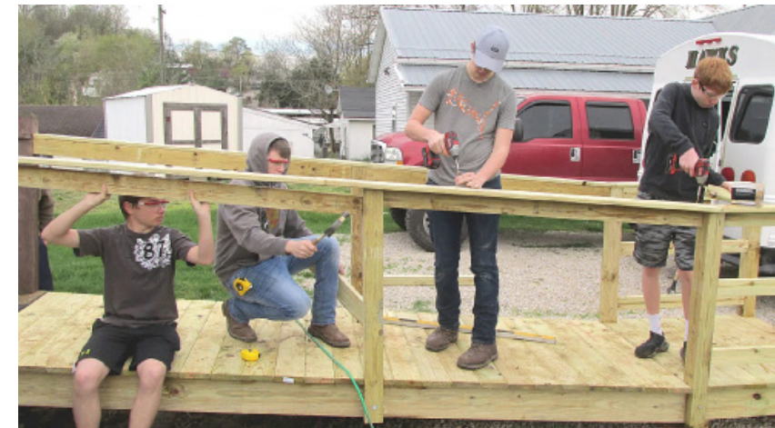
Trade students constructing an access ramp
